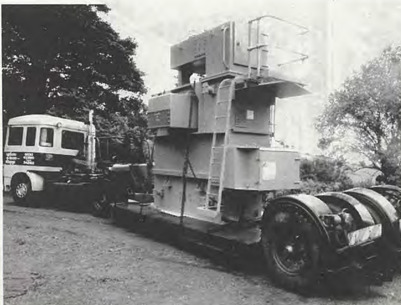
New equipment arrives at Bow Street sub-station
