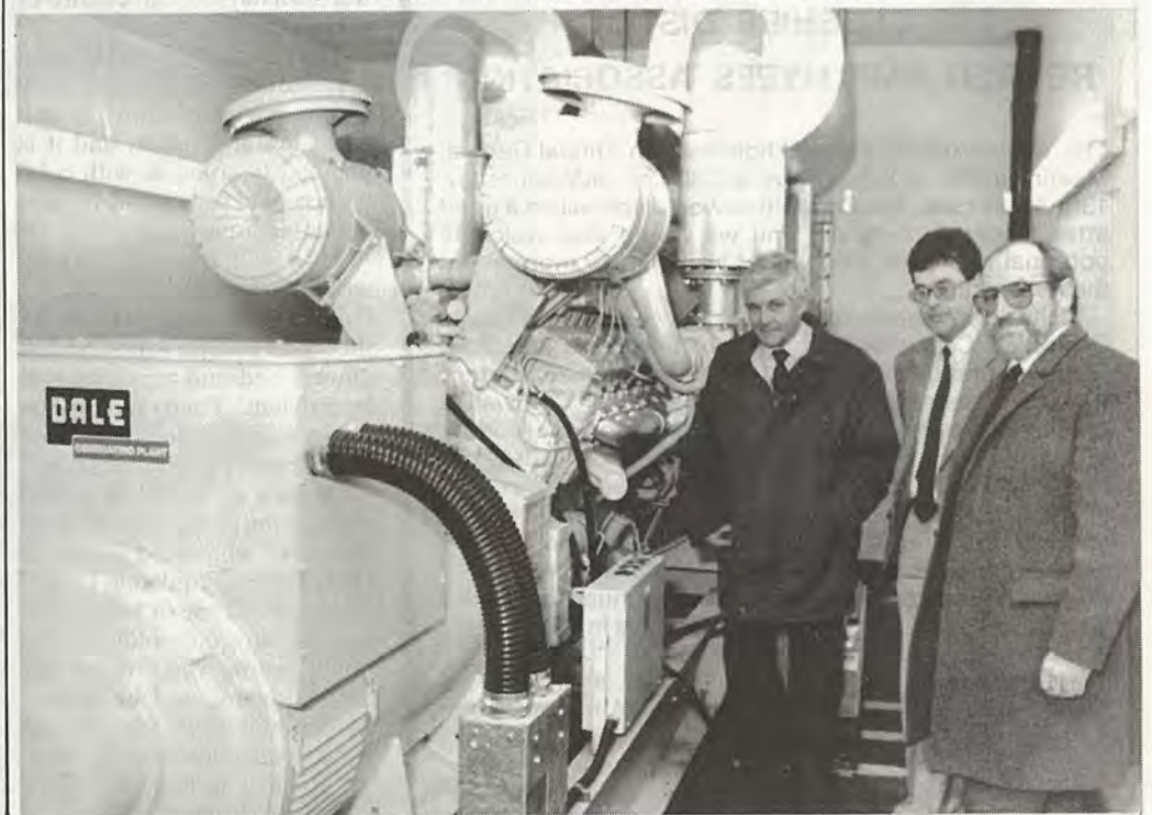
Inspecting the stand-by generator in the new sub-station
